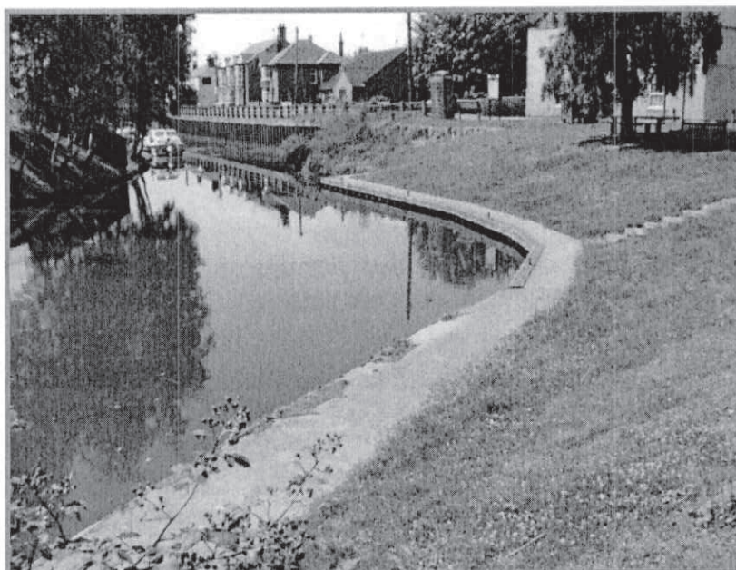
Photo 6: The boat basin, Outwell, Norfolk (application granted)
